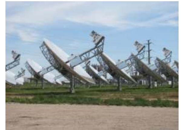
Figure 14. Dish/engine solar field
